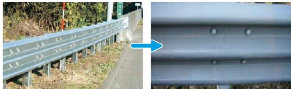
No red rust was observed on its surface even after the lapse of 5 years since construction.
