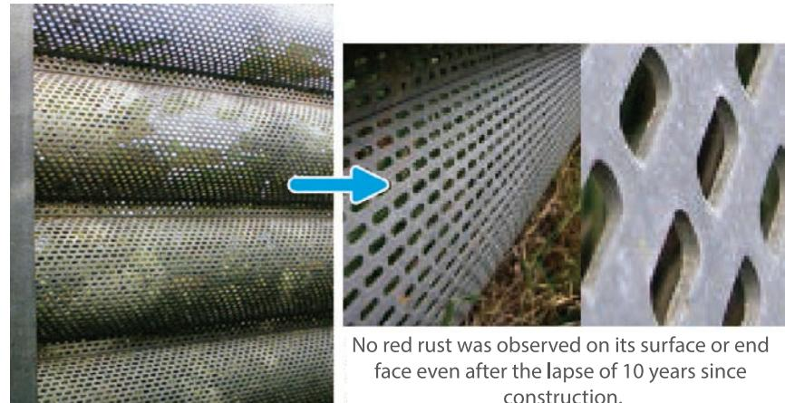
No red rust was observed on its surface or end face even after the lapse of 10 years since construction.
